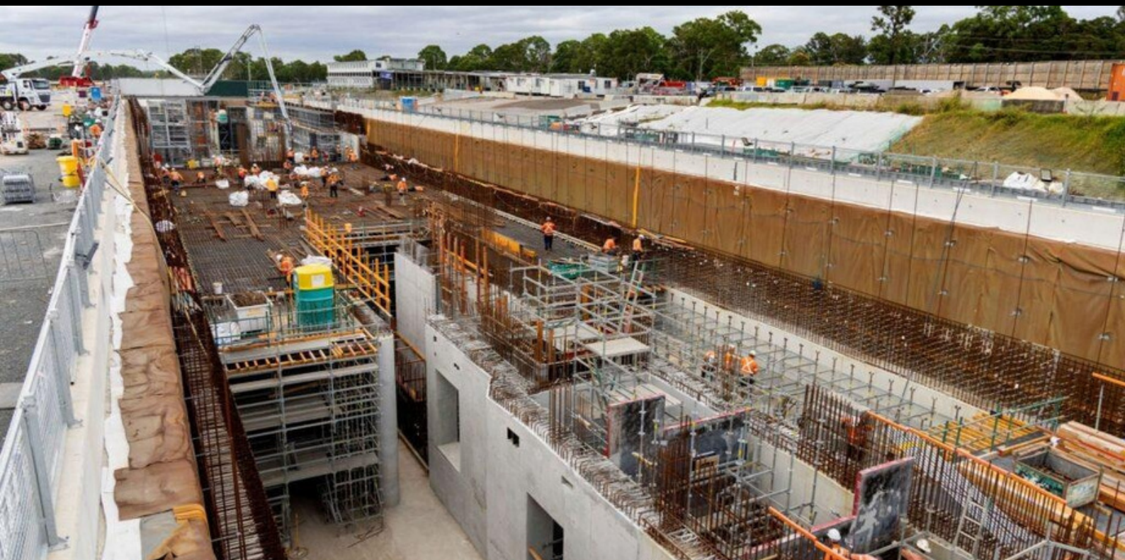
Orchard Hills Station Construction Progress
