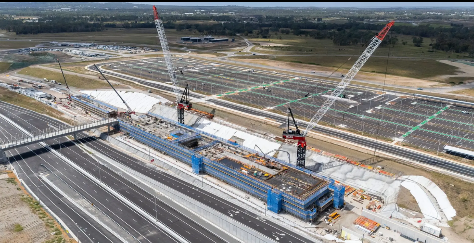
Major Infrastructure and Civil Works
